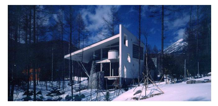
The "Three Walls" concept, which evolves in later works, defines the space within Villa TCG. A stone wall, referencing a stone kiln that once stood on the site, curves in the form of the stream running through the site. Directing the circulation, a red cedar wall flanks the stairs, hallway, and passages to the outdoor. A brick cylinder acts as the third wall, providing service spaces.
