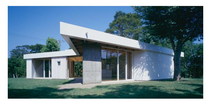
The roof of the Veneer Grid Roof House is made of a triangular veneer grid similar to the triangular paper honeycomb grid of the Nemunoki Children's Art Museum, combined with the aluminium joint of the Hannover pavilion. The roof is supported by prefabricated furniture units and frames the sliding doors, maintaining the flexibility of the space.
