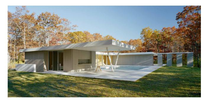
The Sagaponac House is based on the plan of Ludwig Mies van der Rohe's unbuilt Brick Country House (1924), reinterpreted according to program, structure, and site. An improved version of the prefabricated Furniture House system was employed. The corners are reinforced with triangular plywood pieces to bear horizontal and vertical loads and to prevent buckling.
