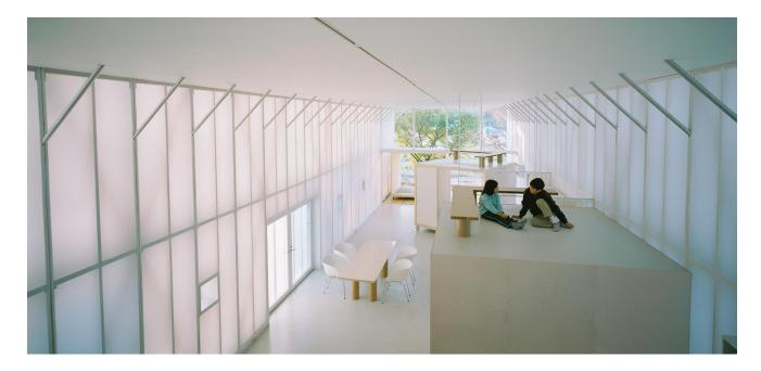
Four freely movable room-boxes on casters in one unique two-storey high room allow three generations of one family to flexibly share a common life as well as individual activities. Diffusing natural light, the two main parallel walls are comprised of two layers of corrugated plastic laid perpendicularly on the outside, an insulation filling of polyethylene strings in clear bubble wrap bags, and a nylon fabric membrane that is velcroed on to the structure on the inside.
