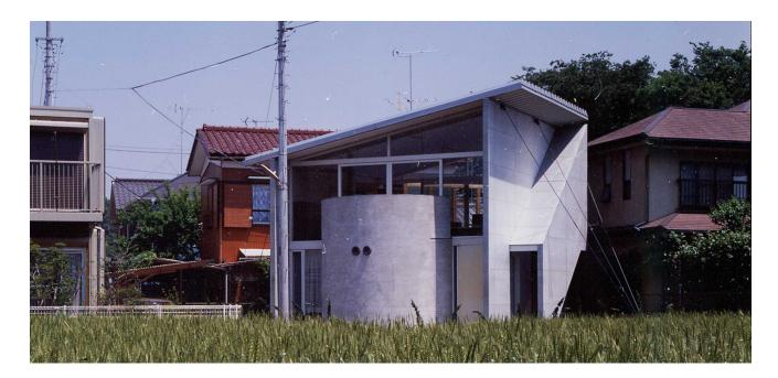
Anticipating future housing development in the area, the house's square plan was rotated 45 degrees to expand views and garden space. In order to reduce time and cost of construction, certain materials were entrusted with two functions. The corrugated steel acts as spanning beams and also as a roof, and the OSB sheets provide shear strength as well as interior finishing.
