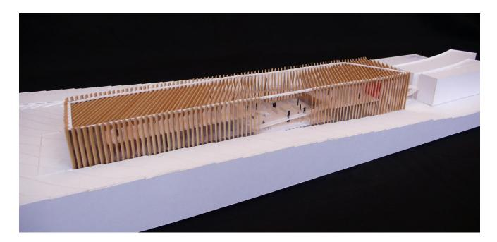
This office building for GC EUROPE headquarters was proposed in Leuven, Belgium. Given that the program requested that all office functions be situated under one roof, an 88m long, 18m wide, 10m tall wooden box-like structure was proposed. The office spaces are arranged in a skip floor configuration, centered around a large atrium space.
