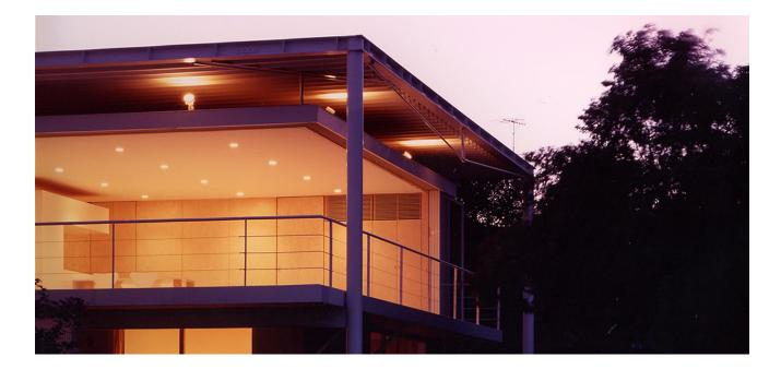
The Furniture House 3 is a further development of the furniture unit system. The second story of the house arranges the furniture units in an L shape to expand the view in one direction. The cantilevering corner of the roof is held up by the double roof which also acts as bracing.
