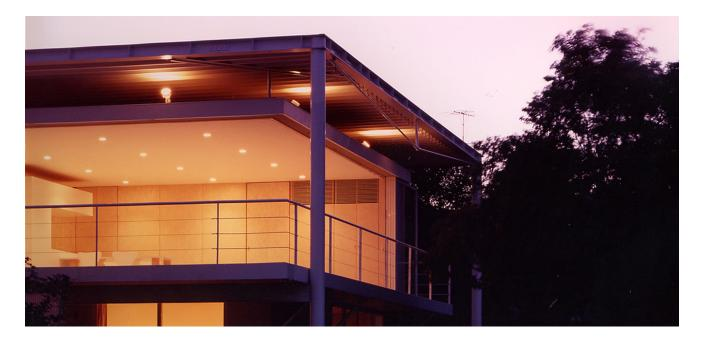
The Furniture House 3 is a further development of the furniture unit system. The second story of the house arranges the furniture units in an L shape to expand the view in one direction. The cantilevering corner of the roof is held up by the double roof which also acts as bracing.
