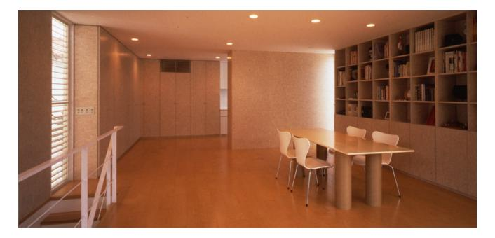
Furniture House 2 is the prototype of a two-story house employing furniture units as structural system. The furniture system used on the first floor is repeated on the second. More furniture units with different functions were developed and combined with "non-furniture" walls to create a system which allowed high flexibility in spatial arrangements.
