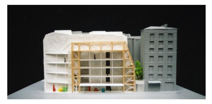
Within the historical "Marais" district of Paris, this apartment building sits on a narrow site flanking an existing fire wall. To minimize disturbance to the wall and to maximize transparency, an independent wooden frame structure was designed to support the suspended floor plates. The openness and flexibility of space is a reaction to the changing lifestyle and working style of Parisians.
