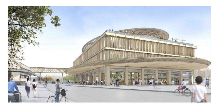
This is a new office building and a showroom of Team7 Company in Austria, which manufactures furniture made only from solid wood. It is a four storied wooden building, and the roof of the penthouse on the top floor is a wooden truss, inspired by the shape of legs this company designs for wooden side tables.
