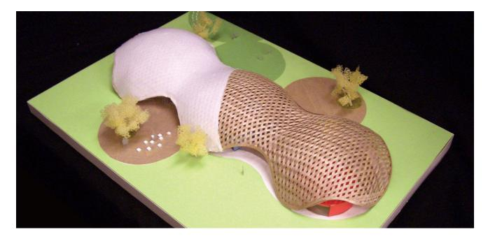
More than one third of the land of the Czech Republic is covered with forests, and we started to think to a kindergarten that can feel the warmth of timber. The design concept became a combination of grid shell domes made of Czech timber. The grid shell creates the dynamic roof, which covers the entire space and the opening within the grid lets the sunlight go through. The light through the transparent insulation becomes gentle and makes a warm atmosphere within the interior spaces.
