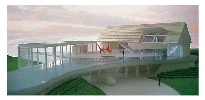
This residence is designed to meet the special conditions of its vast, undulating site opening up to the Atlantic Ocean. Therefore the first floor outline follows the topographic contour of the site, and the second floor features a pool, of which the water surface creates a visual continuity to the ocean. The third floor is lifted up particularly high in the site to obtain extensive views.
