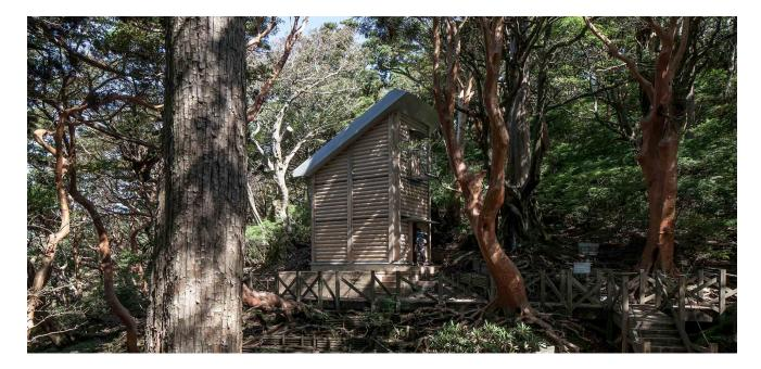
Mountain hut built in the National park of Yakushima Island. The hut was rebuilt on the foundation of the previous dilapidated old hut taken down. The walls allow light to pour inside, by using transparent tubes in-between paper tube. There tubes can be easily replaced if damaged overtime within the harsh environment of the mountains.
