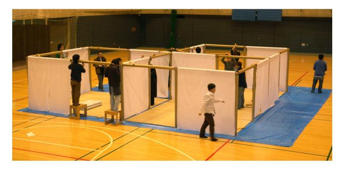
The new Paper Partition System was invented to improve the previous systems. This new system composed of columns and beams is made by paper tubes which are easier and cheaper to acquire in an emergency. The partition can be constructed without using any nails in only 30 minutes. In this system, it is not necessary to stock materials, and it can be easily built by anyone.
