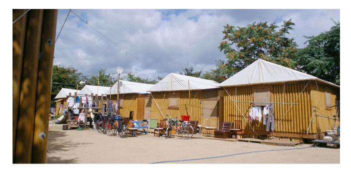
The design criteria for the temporary housing for the Kobe Earthquake victims called for an inexpensive structure that could be built by anyone, with satisfactory insulation and acceptable appearance, that would be easy to dismantle and recycle afterwards. The solution was a kind of log-house cabin with a foundation of sand-filled beer crates, walls of paper tubes, and a roof and ceiling made of tent membranes.
