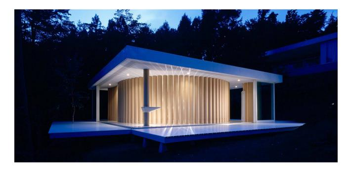
The first permanent paper tube structure, the Paper House is organized on a  $10 \times 10$  meter plan with 110 paper tube columns arranged in an S shape, creating various inside and outside spaces. 80 paper tubes bear the lateral forces and 10 tubes carry the vertical load. When the sliding glass doors open, the horizontal roof over the paper tubes becomes ever prominent, and the interior and exterior become one.
