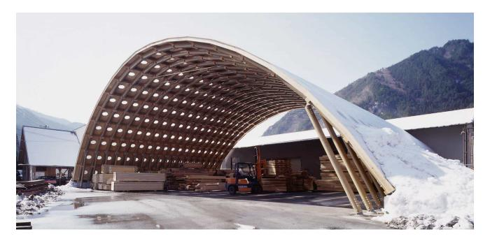
This permanent paper shelter was designed for a contractor of wooden houses. Because paper tubes cannot be bent, a segmented arch was created with wooden joints. Lateral stability was accomplished through the use of structural plywood boards instead of metal bracing, each punched with the maximum allowable aperture to let in light. Finally, a layer of corrugated polycarbonate was used as exterior cladding.
