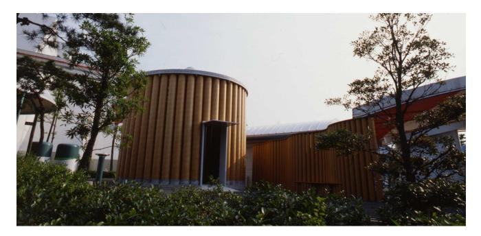
Created for the 1989 Design Expo, the Paper Arbor is comprised of 48 water-proofed paper tubes that fit into a pre-cast concrete base. A compression ring at the top of the structure stabilized the tubes and anchored a tensile fabric roof. The small gaps between the tubes allowed wind and light to pass through softly, and at night, the Arbor turned into a lamp with 48 strips of light.
