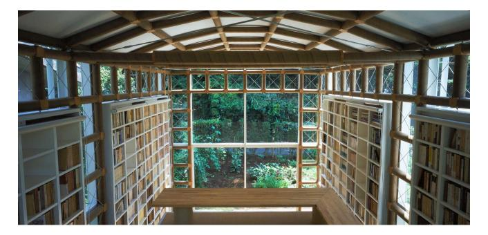
The paper tube truss of the East Gate of the Odawara Festival was again employed in the Library of a Poet, but here wood joints replaced steel. Prefabricated, full-height bookshelves, equipped with insulation and exterior finish, were fixed to the ground and stand independently of the structure with strength to absorb wind loads.
