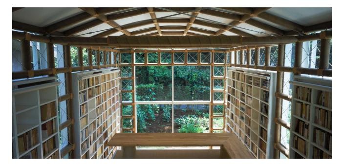
The paper tube truss of the East Gate of the Odawara Festival was again employed in the Library of a Poet, but here wood joints replaced steel. Prefabricated, full-height bookshelves, equipped with insulation and exterior finish, were fixed to the ground and stand independently of the structure with strength to absorb wind loads.
