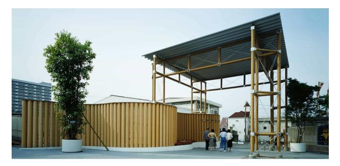
Because building codes did not require official permits for the construction of gates, the East Gate of the Odawara Festival was able to become a real paper tube structure. In this Vierendeel gate structure, the primary structural members were the paper tubes, which were connected by steel joints and braced by steel tensile members. Post-tensioned members also ran within the tubes, further stabilizing the structure.
