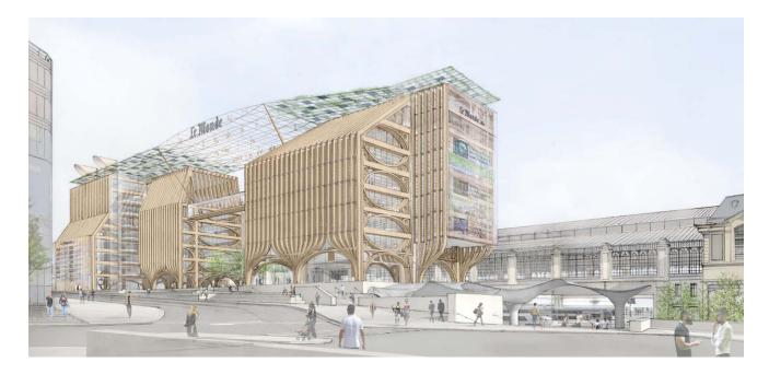
A design competition for the new headquarters for the French media company, Le Monde. Configuration of the building was driven by structural restrictions of the site which is located above the train tracks, as well as zoning regulations. A light weight timber structure in combination with various renewable energy methods were proposed.
