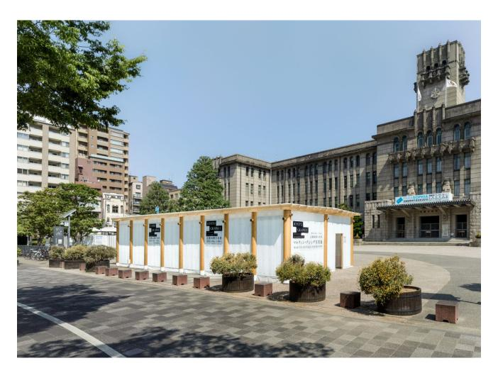
A temporary paper tube pavilion designed for Martin Gusinde Photo Exhibition at Kyotographie International Photo Festival was built in the middle of the open square at Kyoto City Hall. 27 columns made of paper tubes with a diameter of 330mm were used to make the exhibition space. It was built by volunteers mainly from Kyoto University of Art and Design and the photo exhibition was held for one month.
