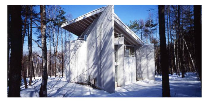
Walls facing east and west define the space of Villa Torii, harmonizing interior and exterior by inviting the sun and wind to pass through freely. Laminated wood girders are fastened on top of these two main walls and braced by tension cables running to the ground. The space within is further defined by curved, freestanding masonry walls.
