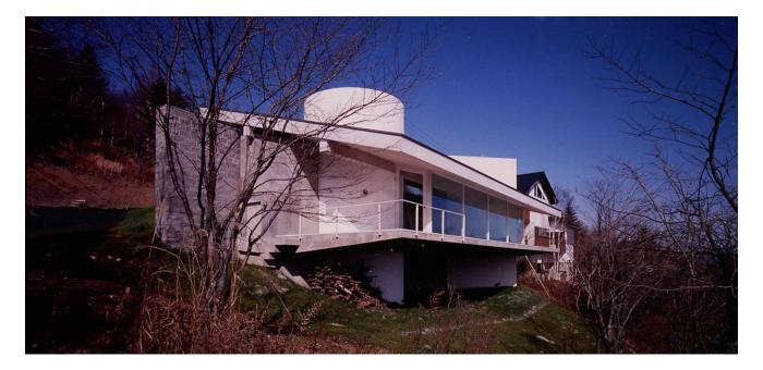
With intentions of framing the extraordinary mountain landscape, a rough stone wall was placed parallel to the street to contrast the view upon approach and entry. A circular core containing wet spaces and a square core with bedrooms provide the main structure, allowing a cantilevering floor to thrust out towards the mountains, offering unobstructed panoramic scenery.
