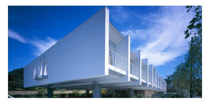
The structure of this company dormitory is organized by two parallel Vierendeel trusses that sit on eight columns, and a series of perpendicular secondary trusses. Within this rhythm of walls are 23 single apartments and a guest room, which float above the openable common area and parking below.
