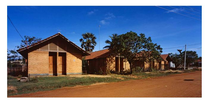
In order to help the victims of the tsunami in 2004, 80 houses and a mosque were planned to recreate the village of Kirinda in the southern part of Sri Lanka. The houses' structure mainly consists of inexpensive and locally produced compressed earth blocks and furniture units made of wood from local rubber trees, an experimental but locally available building material.
