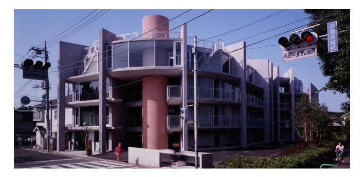
To create a sense of openness in the Housing at Shakujii Park, the axial shear wall was eliminated by arranging nine reinforced concrete walls like dominoes in an "S" shape that were connected with horizontal floor slabs, distributing lateral forces throughout the building. This arrangement of walls enabled an overall structural system while maintaining independence of the apartement units, each placed between two walls.
