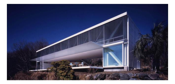
The main intention for the design of the Picture Window House was to frame the panoramic view while maintaining the flow of the mountain to the sea. The whole upper story works as a truss spanning 20 meters, creating a completely open and columnless space below. The  $20m \times 2.5m$  "picture window" gives an unobstructed view to the ocean.
