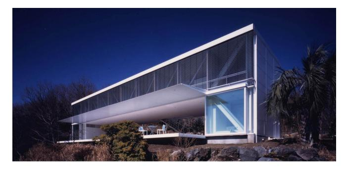
The main intention for the design of the Picture Window House was to frame the panoramic view while maintaining the flow of the mountain to the sea. The whole upper story works as a truss spanning 20 meters, creating a completely open and columnless space below. The  $20 \, \mathrm{m} \times 2.5 \, \mathrm{m}$  "picture window" gives an unobstructed view to the ocean.
