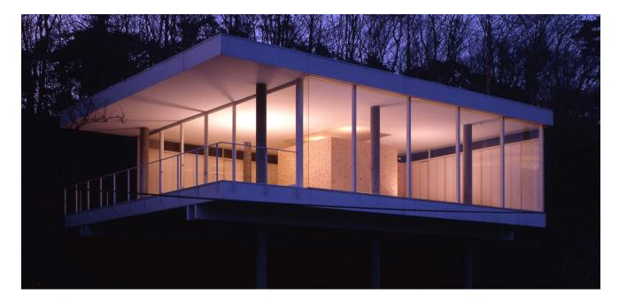
Although the sloping site is as steep as 45 degrees in some locations, extra budget could not be alotted for the foundation as a low-cost structure was requested. To maintain privacy the floor was lifted off the ground, with long pre-cast concrete piles used as columns to directly support both floor and roof. While open to spectacular views to the south and east, the north and west sides were glazed with a double layer of translucent polycarbonate panels insulated with granulated urethane foam.
