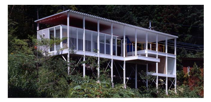
Built in a region with heavy snowfall, the second Case Study House sought to separate roof and ceiling. In order to take the snow loads, the roof was reduced to a single sheet of corrugated steel hovering above the entire house. The separated ceiling is freed from the effects of deflection due to snow loads, and the factor of loads is close to zero.
