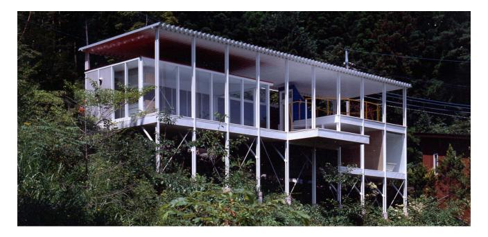
Built in a region with heavy snowfall, the second Case Study House sought to separate roof and ceiling. In order to take the snow loads, the roof was reduced to a single sheet of corrugated steel hovering above the entire house. The separated ceiling is freed from the effects of deflection due to snow loads, and the factor of loads is close to zero.
