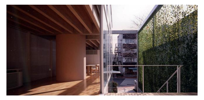
The rectangular plan of the House for a Dentist is divided lengthwise into a southern outdoor space and a northern interior volume. Due to poor soil conditions that would have required an expensive pile foundation, the building was made as light as possible instead. The house is structurally composed of two concrete walls, timber floors and a stabilizing core. An ivy screen to the south ensures privacy while preserving ventilation and passage of natural sunlight.
