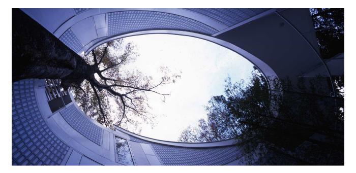
Inherently a three-story row-house complex, the Hanegi Forest succeeded in preserving every existing tree on the site. To ensure that the floors remained rigid even with openings to bring in light to the ground level, an equilateral triangle structural grid was conceived. The pilotis of the first floor open space give the impression of walking in a forest, while the mirror glass of the entrance stairwells minimizes its existence while multiplying the image of the forest.
