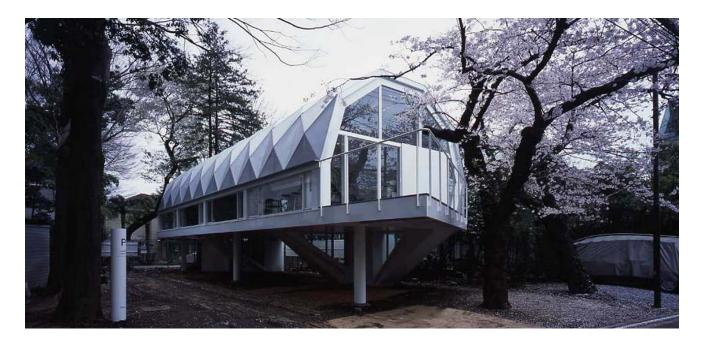
In order to guarantee sufficient parking space at the ground level, the one story high steel frame structure of the annex is lifted up over the ground. The four entry stairs extend out to all directions, simultaneously acting as bracing. The annex's most prominent feature is its self-supporting arched roof made of a folded plate structure.
