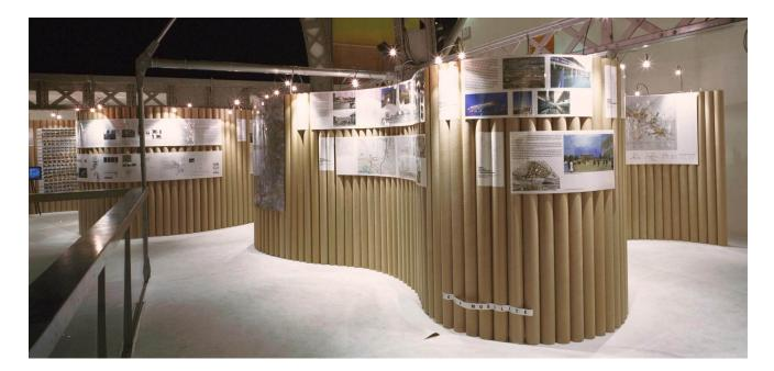
The design for this exhibition required a system which would be flexible and adjustable to travel from one location to another and would provide wall display space of undefined size as well as three spaces for video shows. The wall displays were made of round and square paper-tubes, and for the video spaces aluminium pipes from the previous exhibition were re-used.
