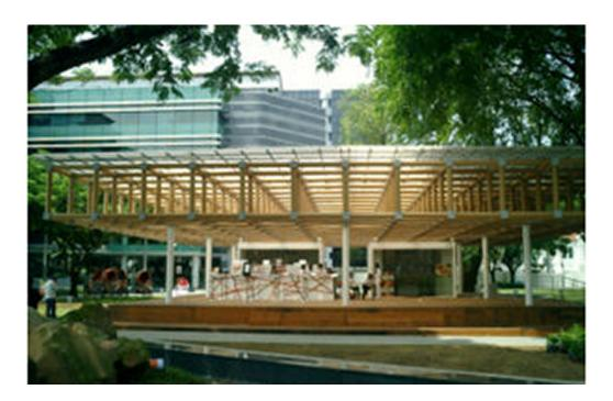
As an information center and press center for the 2006 Singapore Biennale, this is the first space frame structure to be constructed of paper tubes.
