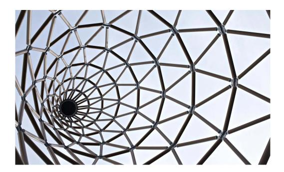
A temporary tower made of paper tubes designed for the London Design Festival. The aims of this project were to challenge the perception of the everyday materials used, by creating dramatic temporary installations outside the Festival Hall. The tower is made from cardboard tubes and articulated by metal joints. The structure is 22m high and became the tallest paper tower in the world. This can be transformed to a permanent structure utilized as an observatory, a green house and a house.
