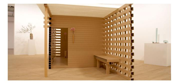
The Paper tea house is made of square paper tubes. Walls are connected by a steel rod and the roof is made of folded paper. The floor and furniture are also made of the same square paper tube profile except the table made of honeycomb cardboard. The prefabrication process of elements allows for very easy assembly and disassembly.
