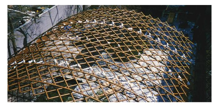
The Paper Arch is made entirely of paper tubes, spanning over the sculpture garden of the MoMA in New York, as a contribution to the experimental architecture exhibition. Unlike the Hannover Pavilion, the lateral spanning arches of this structure were able to be made of paper as well, resulting in a pure paper architecture.
