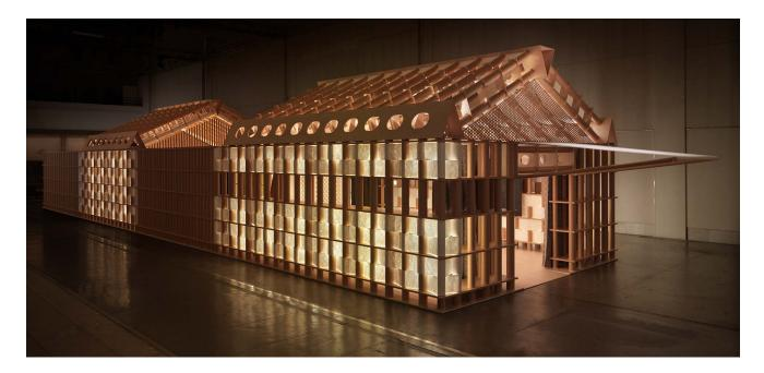
The concept of the pavilion was to create a nomadic exhibition structure easy to assemble and disassemble; all the structure is made of 4 different diameters of paper tubes and connected with wood standard panels to create the horizontal elements. This structure using standard prefab elements also permits to create many different shapes according to future site condition. In order to reduce the volumes for shipping, it is possible to nest the 4 different diameters of paper tubes.
