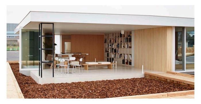
Instead of being supported by conventional columns and walls, this "Furniture House" is supported structurally by the furniture itself, creating a spacious and simple space which eliminates all extraneous and redundant elements. Furthermore, the furniture and unit details will be standardized to Muji storage compartment modules, bringing the utmost simplicity to the "Furniture House" design.
