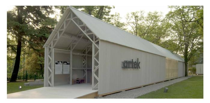
UPM developed a new material called "Wood-Plastic Composite" which is self-adhesive label materials made of paper and plastic. Artek asked us to design their pavilion using this material. We used a truss system in this building because of its strength and elastic nature.
