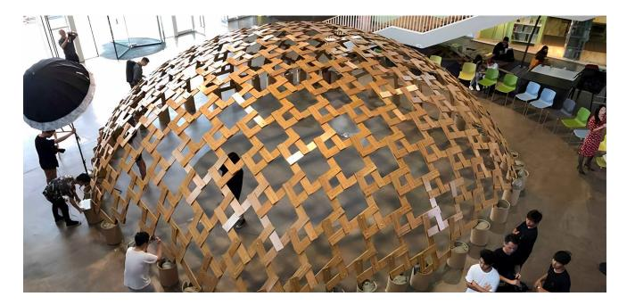
Commonly used as flooring materials in China, bamboo flooring (thickness: 17mm, width: 130mm, length: 1,100mm) with bolt fasteners form a reciprocal frame structure. This dome was collaboratively constructed by Ban laboratory in Keio University and Tongji University.
