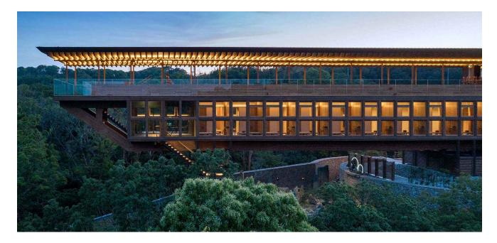
This is a plan of an accommodation facility where guests can experience "zazen" on a small, lush site on Awaji Island. It is located on a ridge of the site and the building has a shorter end of 7.2m and a longer end of 90m. Half of the building is suspended by two steel column bases with wooden vierendeel on the first floor allowing 21m span and the whole second floor will be zazen studio. A cafe with a series of PHP arch frames and a hut are planned for future affiliated use.
