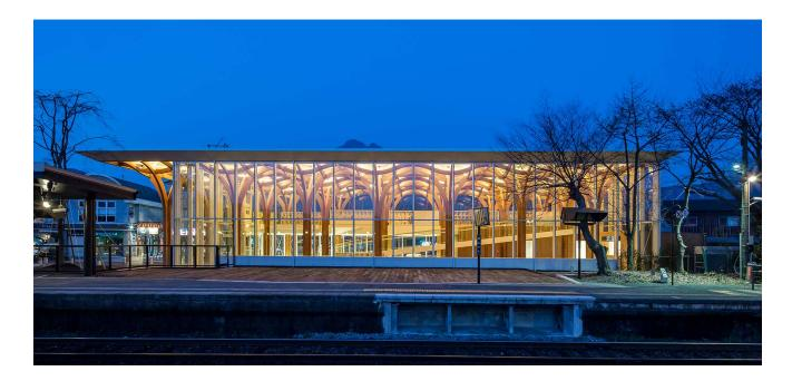
The upper and lower floors are gently connected by a slope in a space where Y-shaped arch columns of laminated timber align. The first floor provides sightseeing information with the railway view of express train "Yufuin no Mori." The slope, overlooking the beautiful mountain range, leads to the "Travel Library" on the second floor storing travel guides in a calm space. The outside is an observation deck where the nearby Mt. Yufu can be enjoyed.
