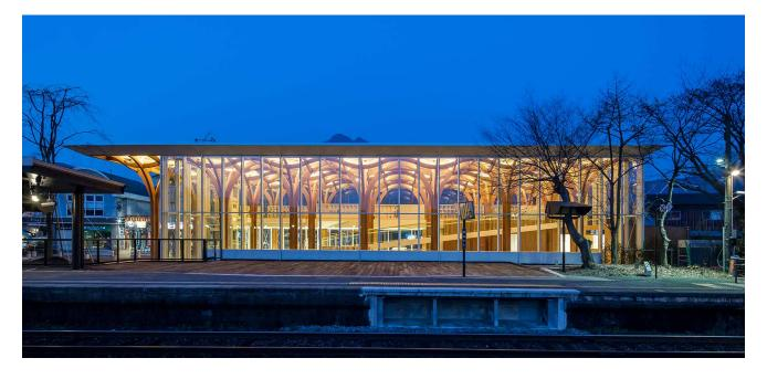
The upper and lower floors are gently connected by a slope in a space where Y-shaped arch columns of laminated timber align. The first floor provides sightseeing information with the railway view of express train "Yufuin no Mori." The slope, overlooking the beautiful mountain range, leads to the "Travel Library" on the second floor storing travel guides in a calm space. The outside is an observation deck where the nearby Mt. Yufu can be enjoyed.
