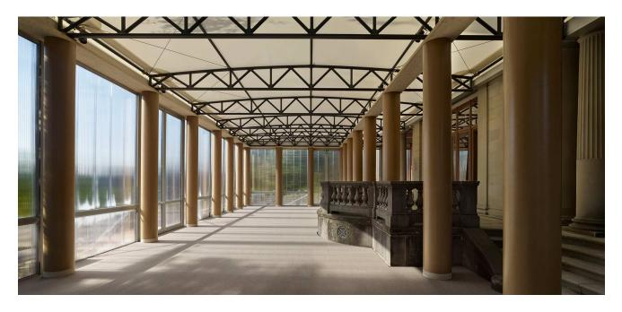
The pavilion is used during the summer months for 3 months then put in storage for the remaining time so two different diameter of paper tubes were used so they can store within each other and minimize necessary storage space. In order to assemble without the use of heavy machinery, polycarbonate exterior panels, carbon-fiber trusses and tent roof was used.
