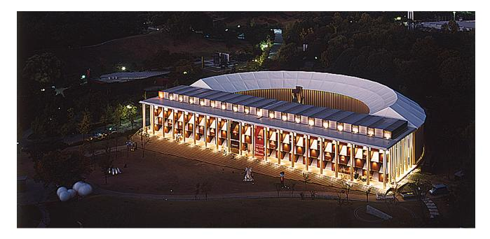
The surrounding forest and circular pass generated the shape of this temporary exhibition pavilion composed of two different spaces. The Container Gallery consists of two parallel, ten meter high walls of shipping containers. The first row of containers is used as exhibition booths while the second row serves as office and storage spaces. The Paper Gallery is organized between two concentric semi-circular walls made of paper tube columns.
