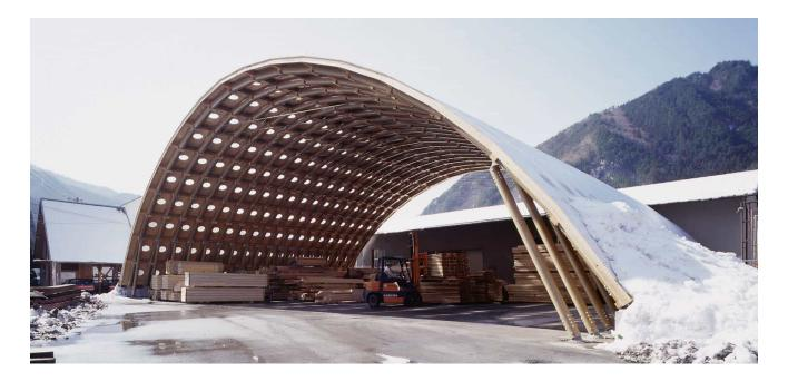
This permanent paper shelter was designed for a contractor of wooden houses. Because paper tubes cannot be bent, a segmented arch was created with wooden joints. Lateral stability was accomplished through the use of structural plywood boards instead of metal bracing, each punched with the maximum allowable aperture to let in light. Finally, a layer of corrugated polycarbonate was used as exterior cladding.
